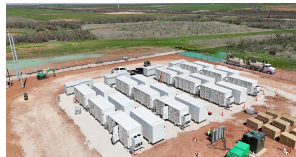
50 MWh of Reuse ESS in Texas being installed in collaboration with a North American partner
